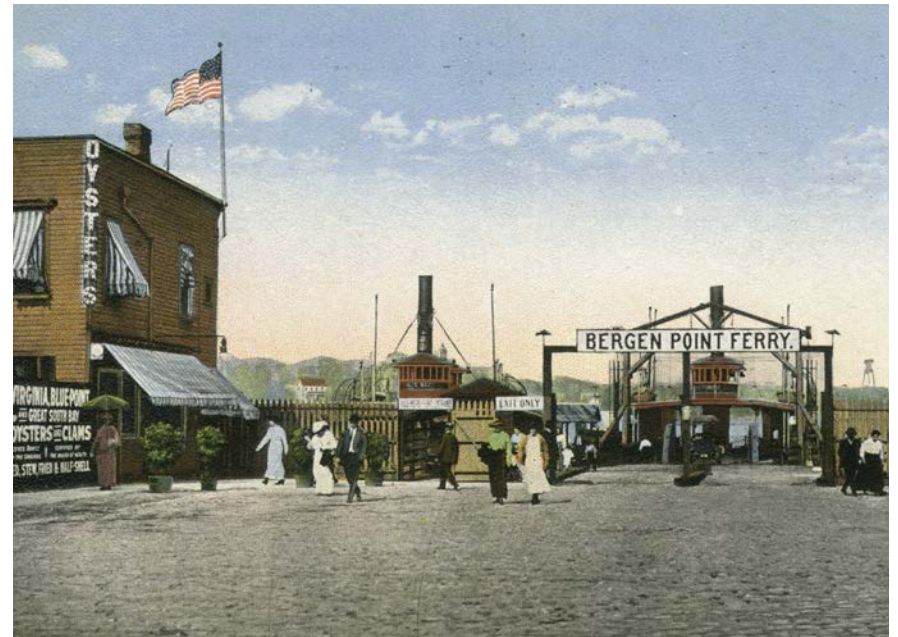
Fig. 45: The Former Bergen Point Ferry (Source: New York Public Library)
