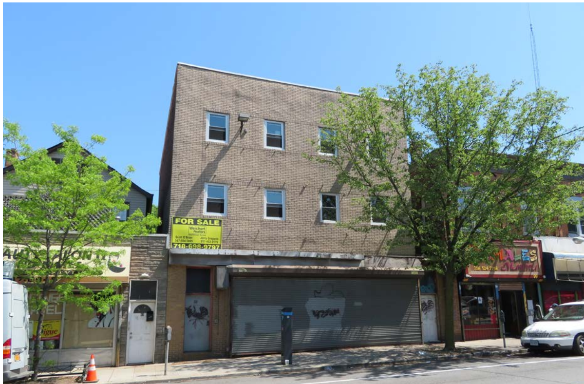
Fig. 69: 97 Port Richmond Avenue
