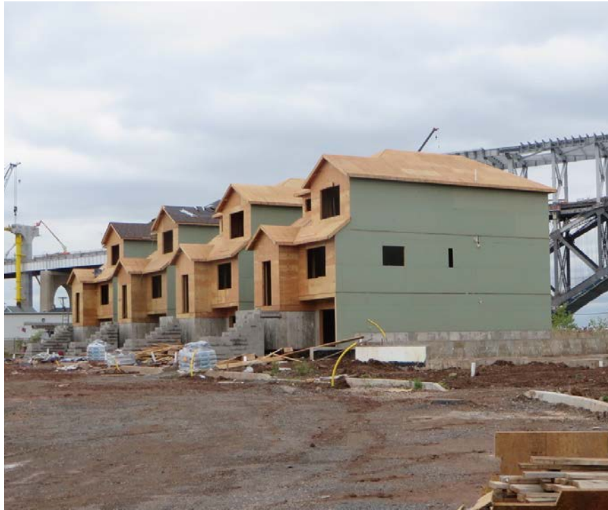
Fig. 54: Two-Family Housing Under Construction at Nicholas Estates
