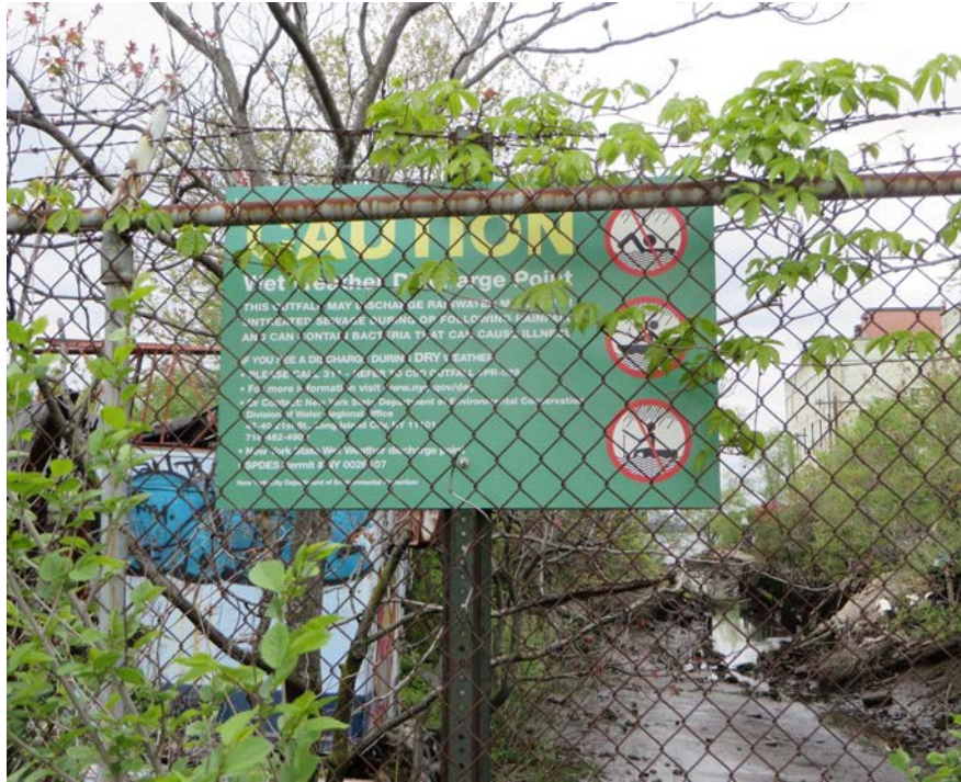
Fig. 4: Combined Sewer Overflow Outfall on Richmond Terrace
