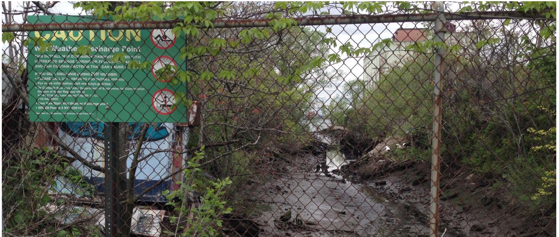
Fig. 47: Combined Sewer Overflow Outfall on Richmond Terrace
