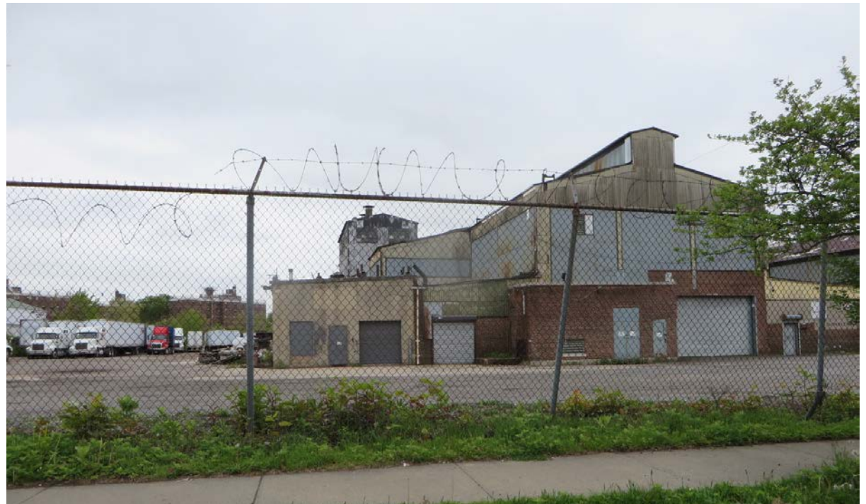
Fig. 61: Davidson Street Industrial Site
